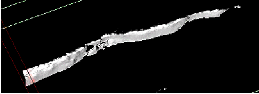
Fig.6. The 3-dimensional image of the formed crack
