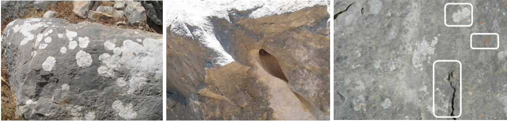
Fig. 1. Sarantapicho: a. Biodecay; b. Cavities' formations; c. Cracks on grey limestone
