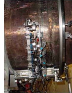
BWR, re-circulation piping weld
