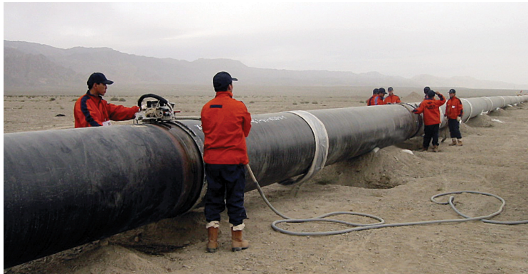
Figure 1 : Photo of typical pipeline AUT operation
