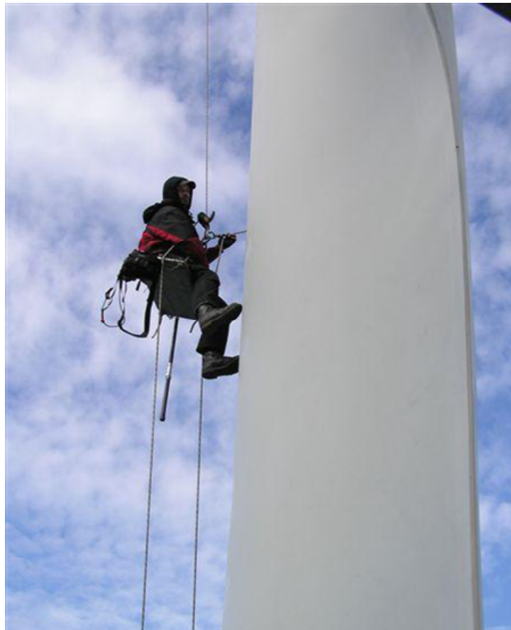
Figure 1. Abseiling personnel inspecting a turbine blade [5].
