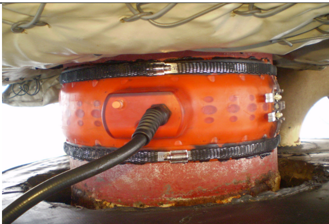
Figure 7 – Installation at casing entrance on an offshore riser.
