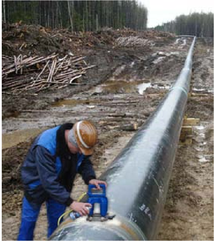
Picture 5. Pipe weld joint inspection using KMU 8/42
