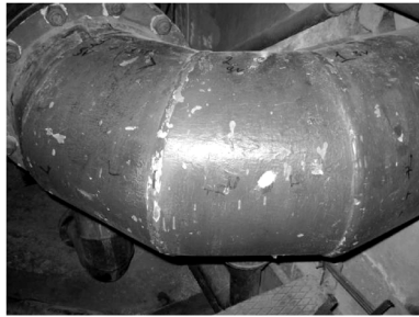
Fig. 1. Part of the pipeline of aluminum alloy SAB-1
